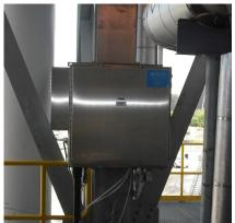
The CEMs is fully self-contained and need only be protected from the sun. Expensive enclosures are remote clean rooms are not required. Just mount it to a post or wall, and you are ready to go.
